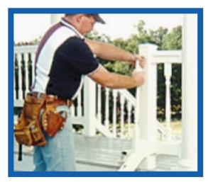
STEP 4: Insert a baluster into the first and last routed hole in bottom rail.
