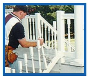
STEP 7: Insert balusters into routed holes.
