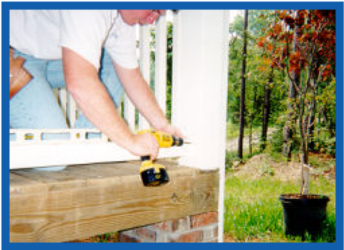
STEP 3: Install bottom rail into opening, level, secure with mounting brackets and screws. TIP: Trim crush block to create horizontal level if necessary.
