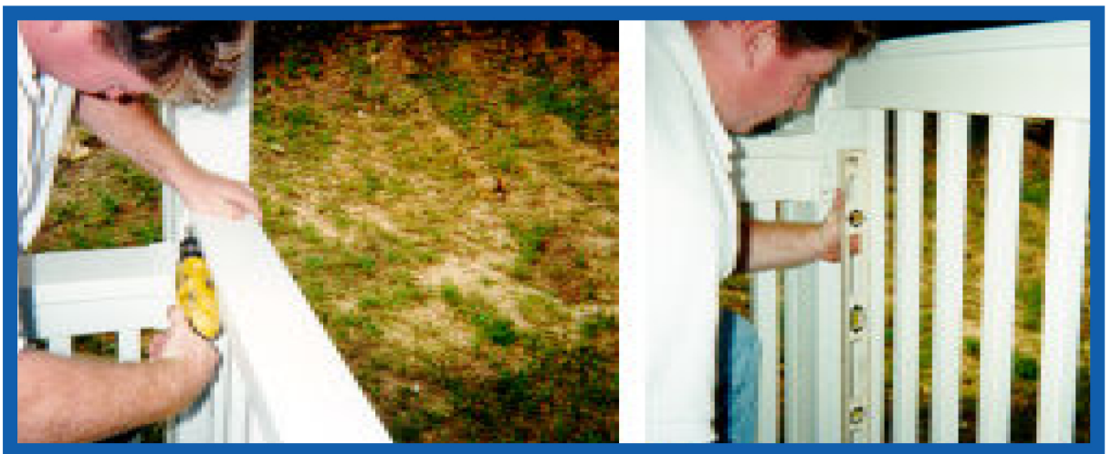
STEP 5: Apply mounting brackets to top rail. Level vertically, and secure with screws.
