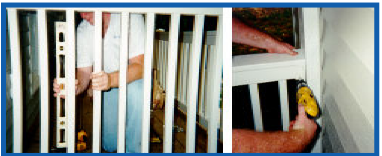
STEP 6: Level balusters and secure rail through bracket with screw. (The hole for this screw is not predrilled).
