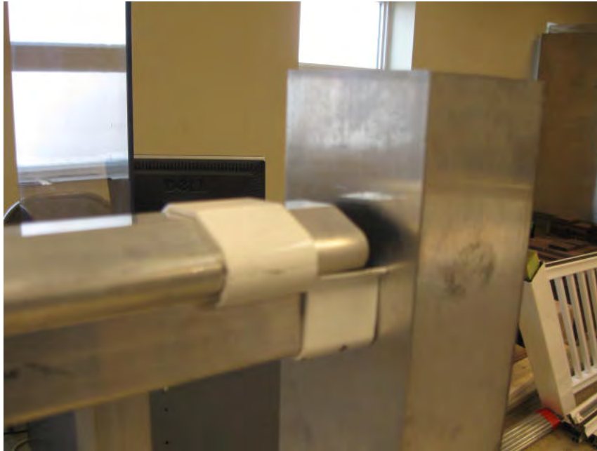
Photo No. 6 Top Rail/Bracket/Post Connection
